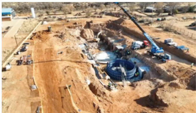
FIGURE 1: May 2024: Breaking ground
