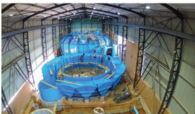
FIGURE 3: July 2025: Three of the modular units visible from the overhead crane
