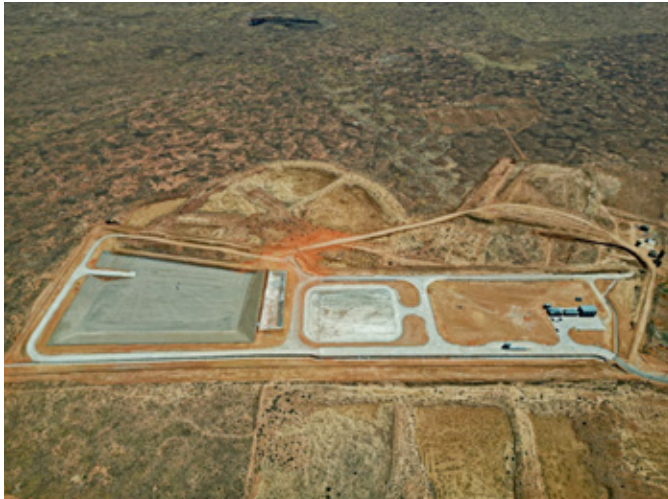
FIGURE 4: Aerial view of completed Weskus Regional Landfill
