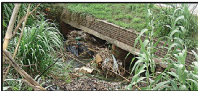
FIGURE 3: Typical type and conditions of urban mayor stormwater drainage systems
