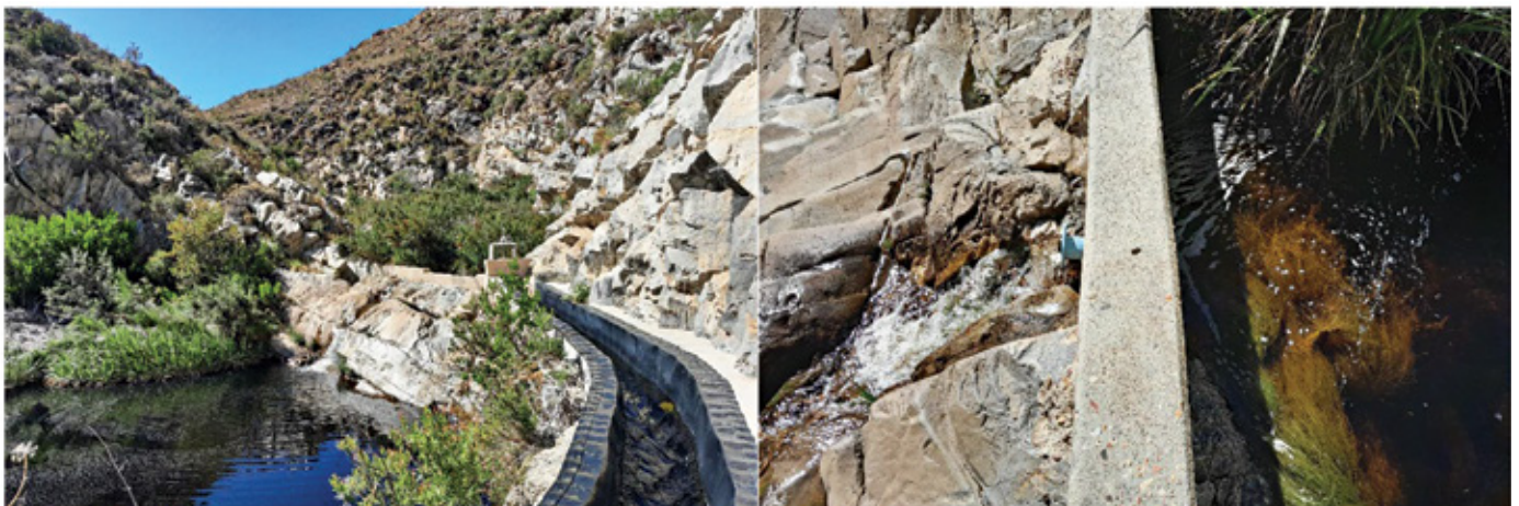
FIGURE 5A AND B: Donkergat weir with diversion canal and 100mm environmental flow pipe
