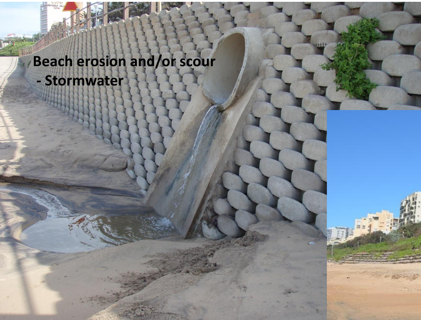
Beach erosion and lowering of the beach elevation seaward of an outlet due to stormwater outflows
