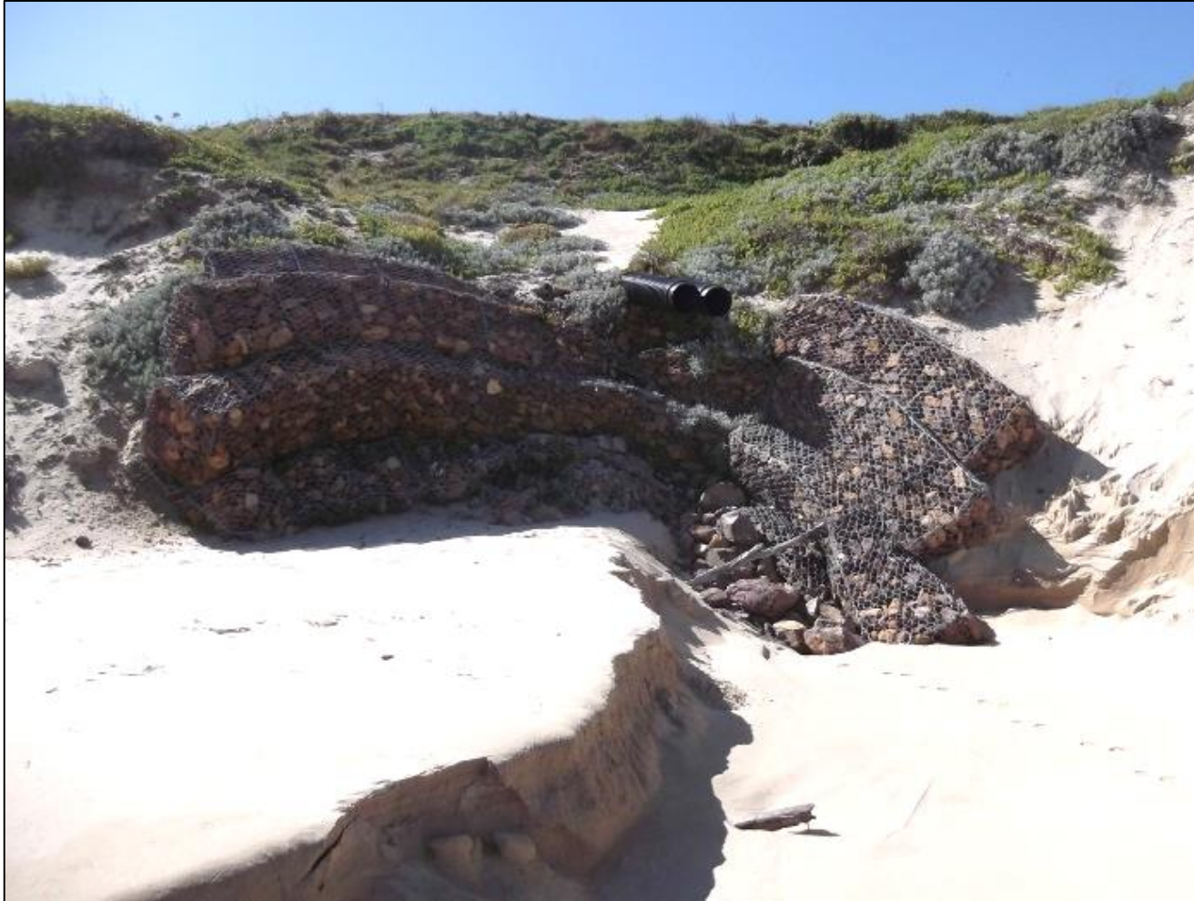
Eroded embankments due to stormwater outflows
