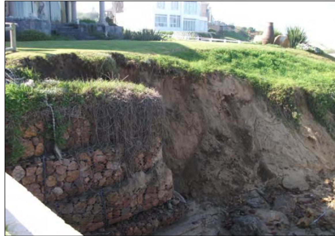
Eroded embankments due to stormwater outflows
