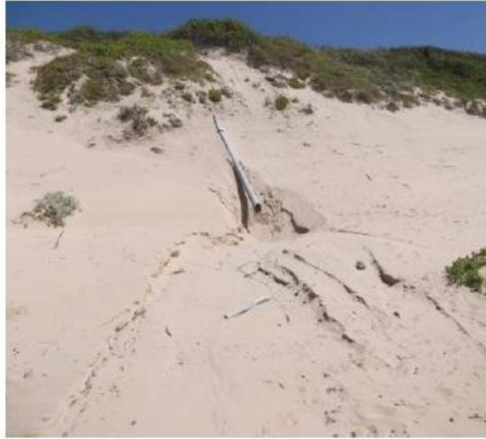
Figure 4.3: Example of damaged outlet in Tergniet area (MVD Consulting Engineers, 2011).
