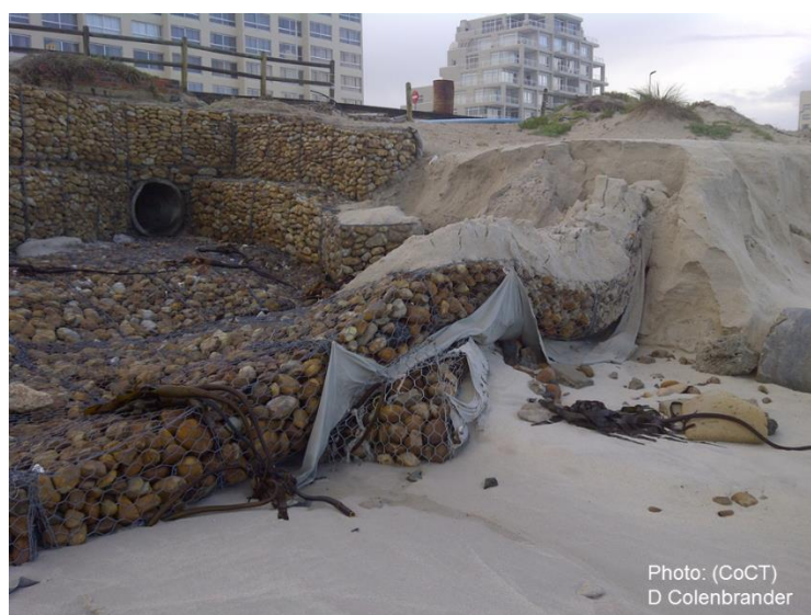
Figure 4.17: Partial failure of a gabion outlet structure
