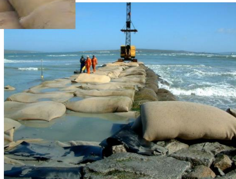
Figure 4.28: Use of the EnviroRock sand bags in South Africa (Kaytech) for general shore protection:
