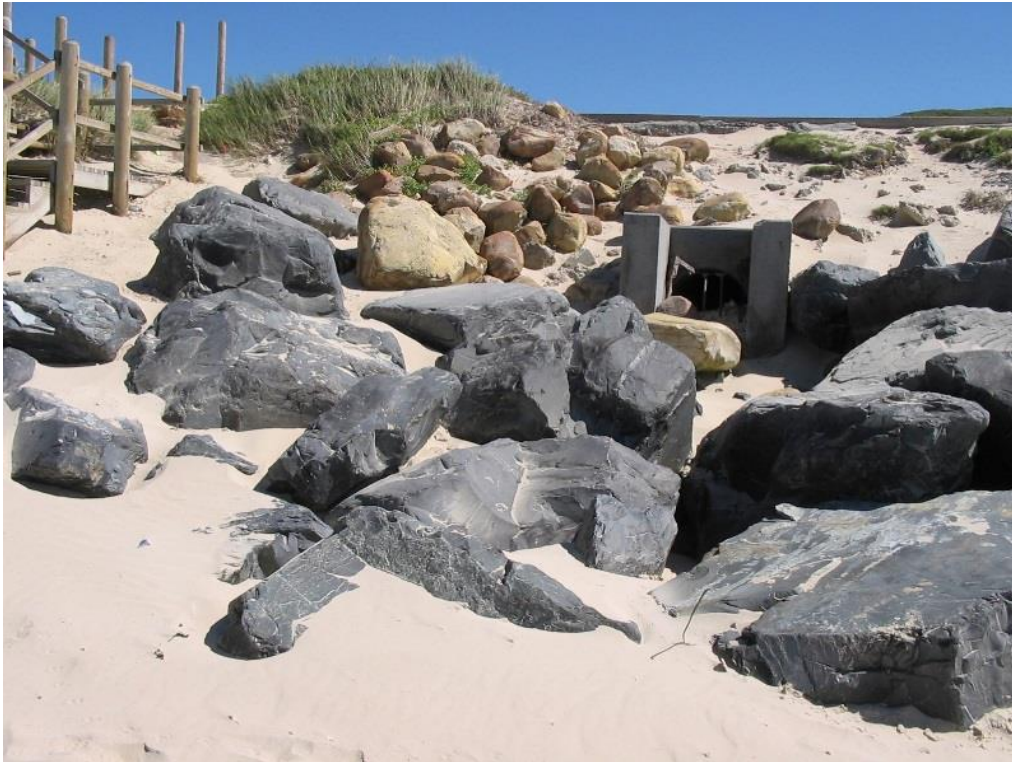
Figure 4.16: Rock armour preventing erosion and scour from both wave action and stormwater runoff. (Photo: A Theron, False Bay)
