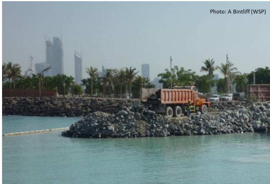
Figure 4.45: An embankment constructed by end tipping (in the Middle East)
