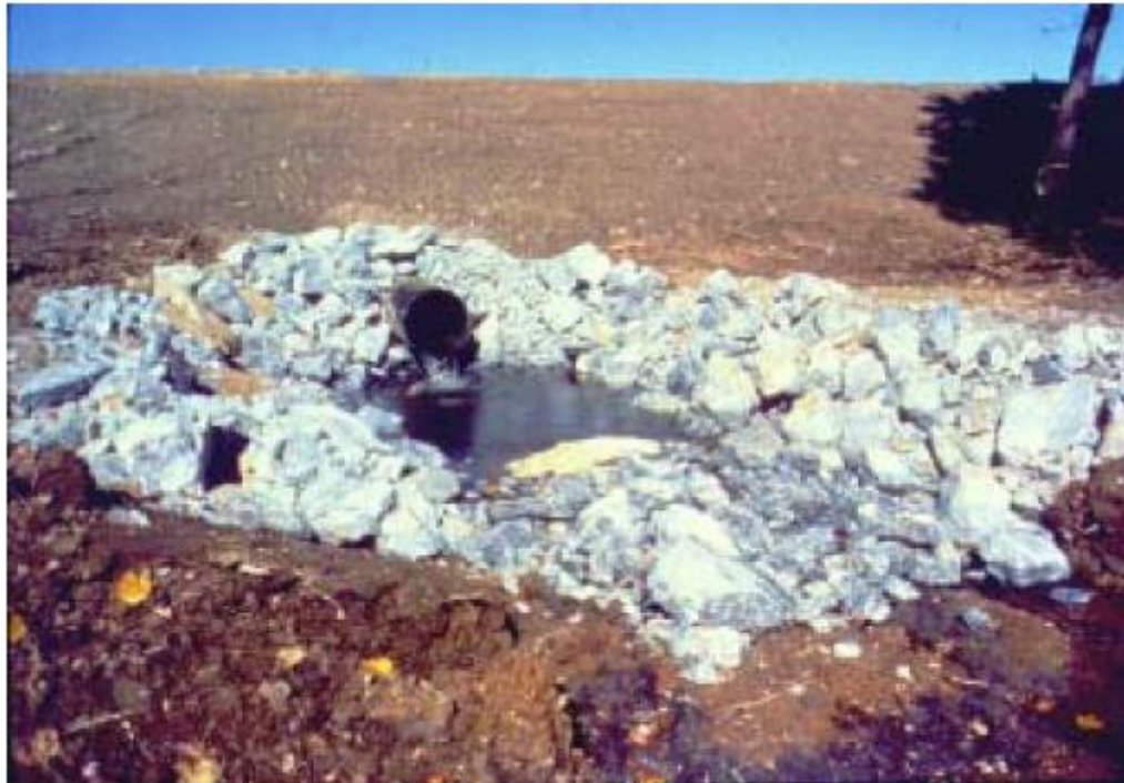
Plate 13-1: Example of riprap at a stormwater outfall
