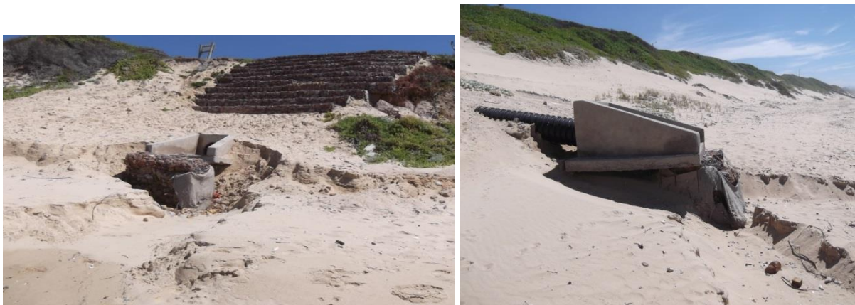
Figure 4.4: Eroded embankments and foundations due to stormwater outflows (Photos: Mossel Bay - Rheeboek, MVD Consulting Engineers, 2011).
