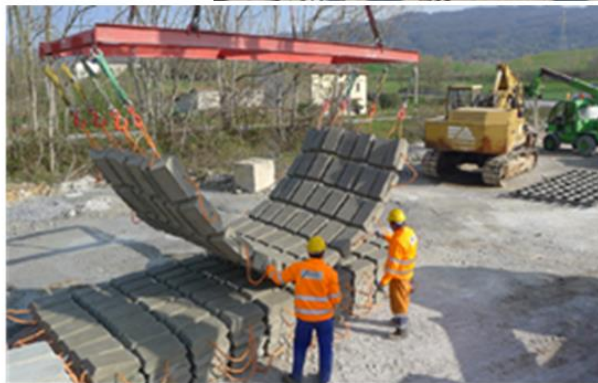
Figure 4.38: Articulated Concrete Block Mattresses by Maccaferri
