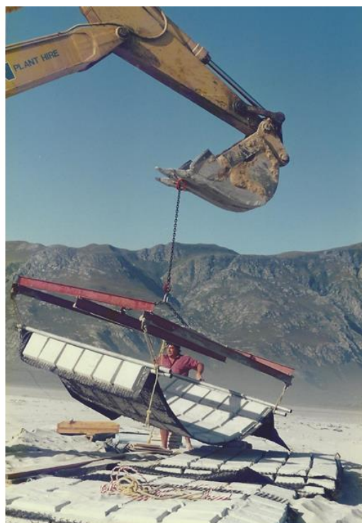
Figure 4.39: Mattress with concrete blocks cast directly onto the geotextile
