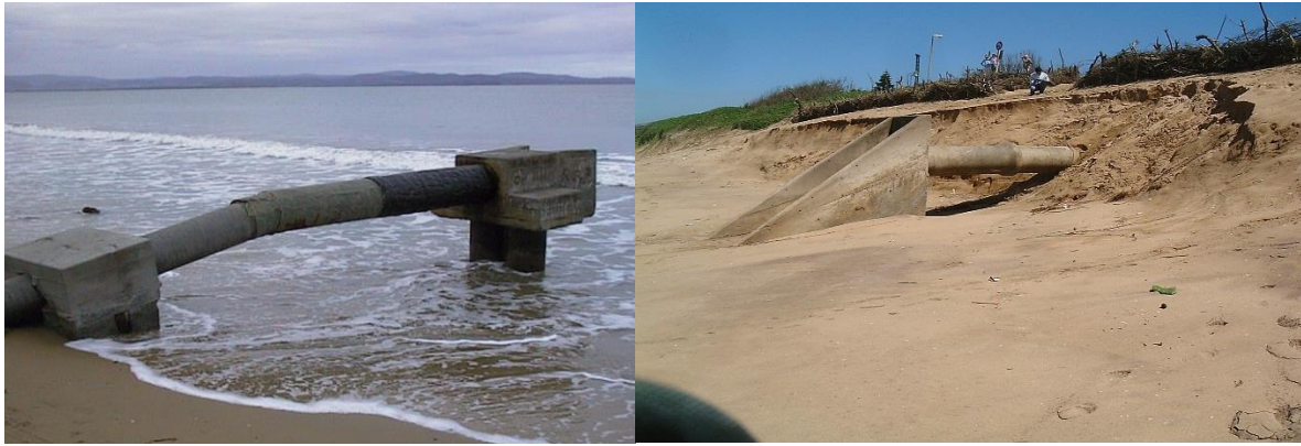
Figure 4.14: Examples of outlet structures that remained intact despite a significant drop in the beach level (photo left: R Cox; photo right: R Kasserchun).
