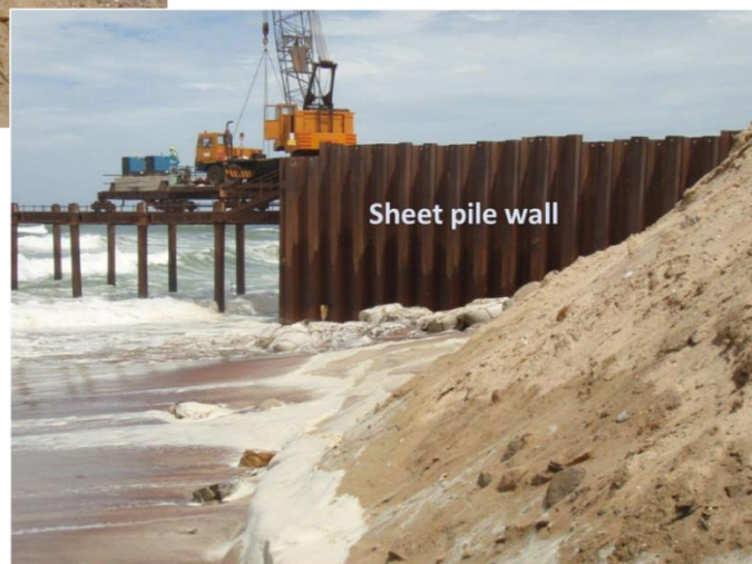
Figure 4.51: Sheet pile wall and jetty for installing a pipe in the surf zone near Swakopmund
