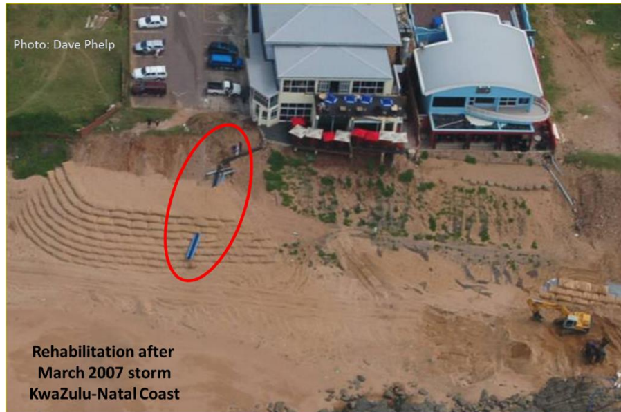
Figure 4.31: Shore protection (using sand bags) on the KwaZulu-Natal coastline, incorporating an outfall
