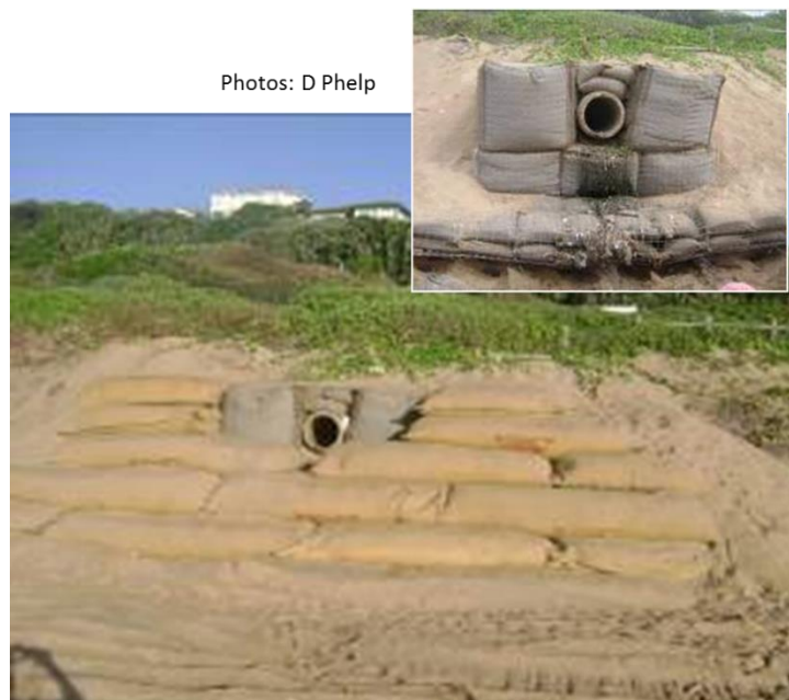
Figure 4.30: A small outfall supported by sand bags (KwaZulu-Natal coastline)
