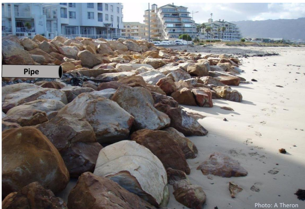
Figure 4.22: Rock revetment protecting an outfall
