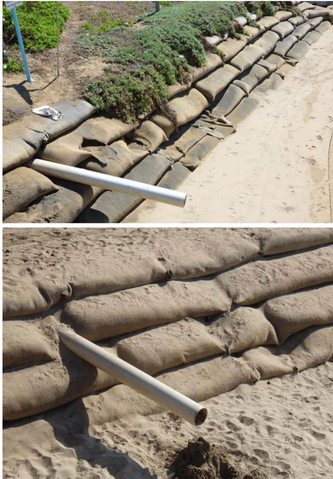
Figure 4.29: Use of the sand bags to support a small outfall along the KwaZulu-Natal coastline
