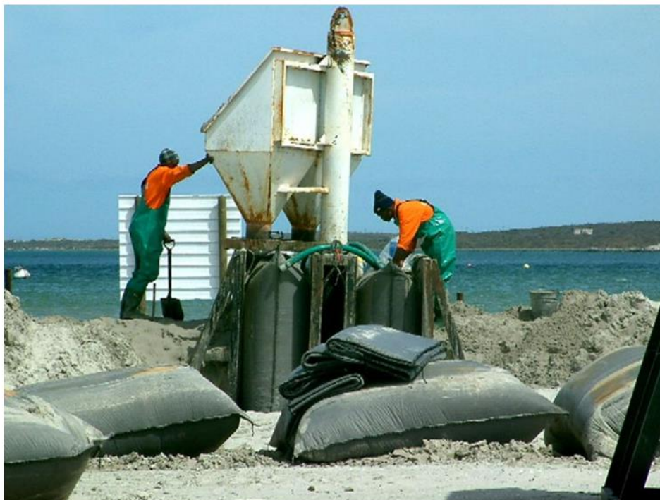
Figure 4.34: Filling sand bags at Langebaan
