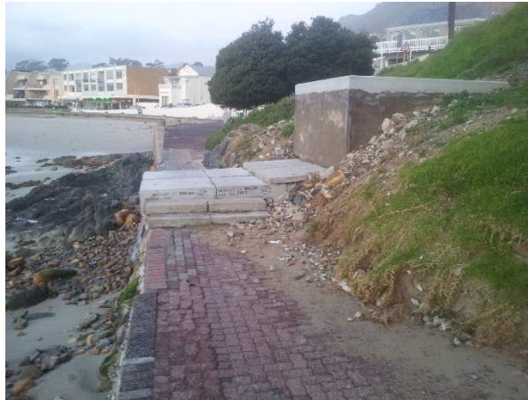
Figure 4.5: Example of a coastal outlet with structure (still incomplete) in which the water is brought down to nearer sea level in a controlled manner (Photo: A Theron).
