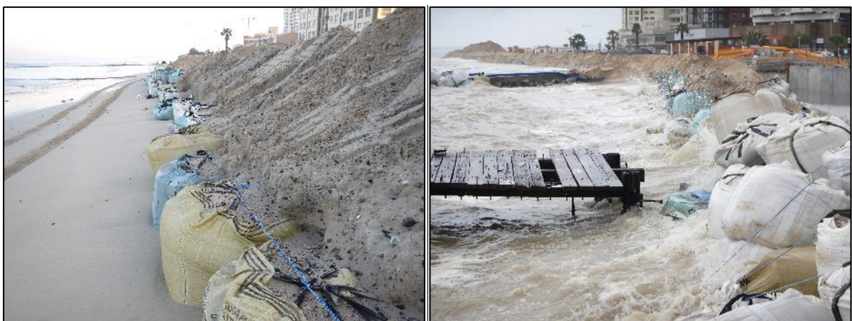
Figure 4.46: Example of coastal construction works protected by a temporary sand wall and sand bag construction. (Photo: A Theron, False Bay, 2016)
