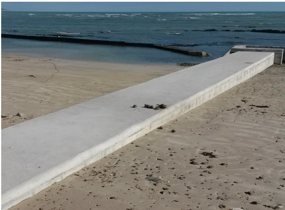
Figure 4.2: Example of an outlet structure hampering public access along a beach (Photo: A Theron)
