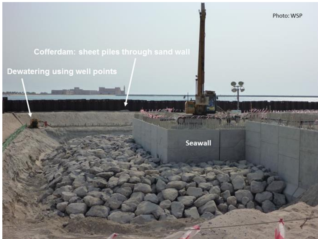
Figure 4.47: A cofferdam with sheet piles and dewatering for large scale construction in the dry in the Middle East
