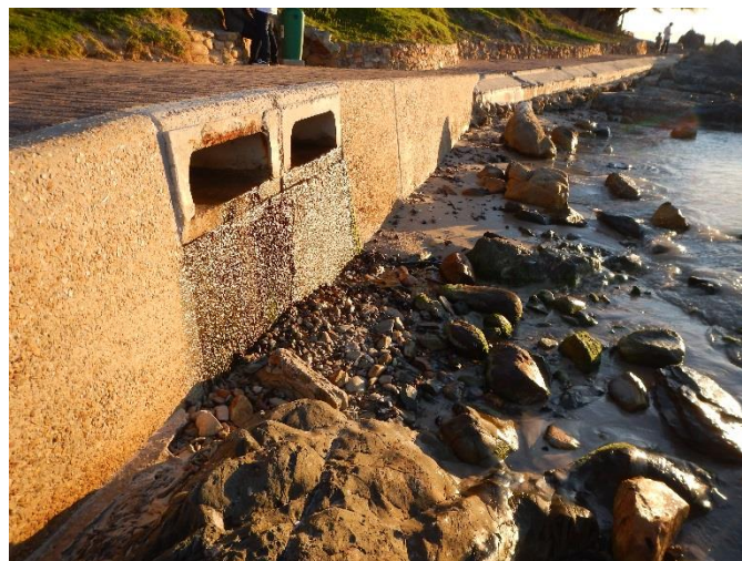
Figure 4.6: Example of an outlet with structure which discharges onto rocks (Photo: A Theron).
