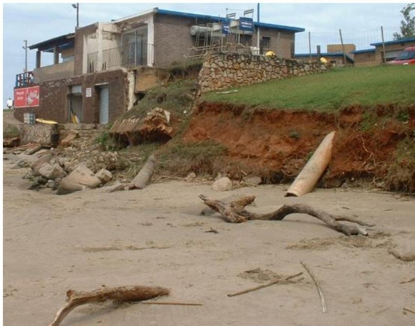
Figure 4.15: Underscouring of an outlet located within reach of storm wave run-up.
