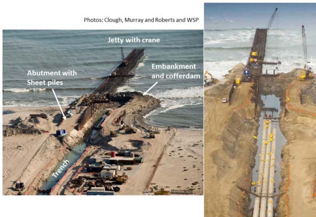
Figure 4.54: Pipelines being placed north of Swakopmund (large scale construction)
