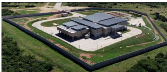
FIGURE 7: Coegakop Water Treatment Works completed.
