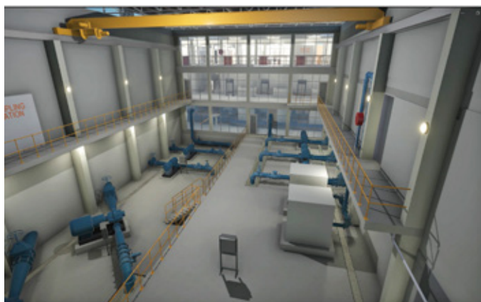
FIGURE 5: Virtual Reality simulation inside Coegakop Water Treatment Works.
