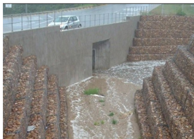
FIGURE 10: Improved inlet configuration (Glentana, Southern Cape)
