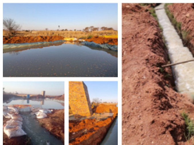
FIGURE 4: Showing constructed channel to direct wastewater to sump and from sump to river
