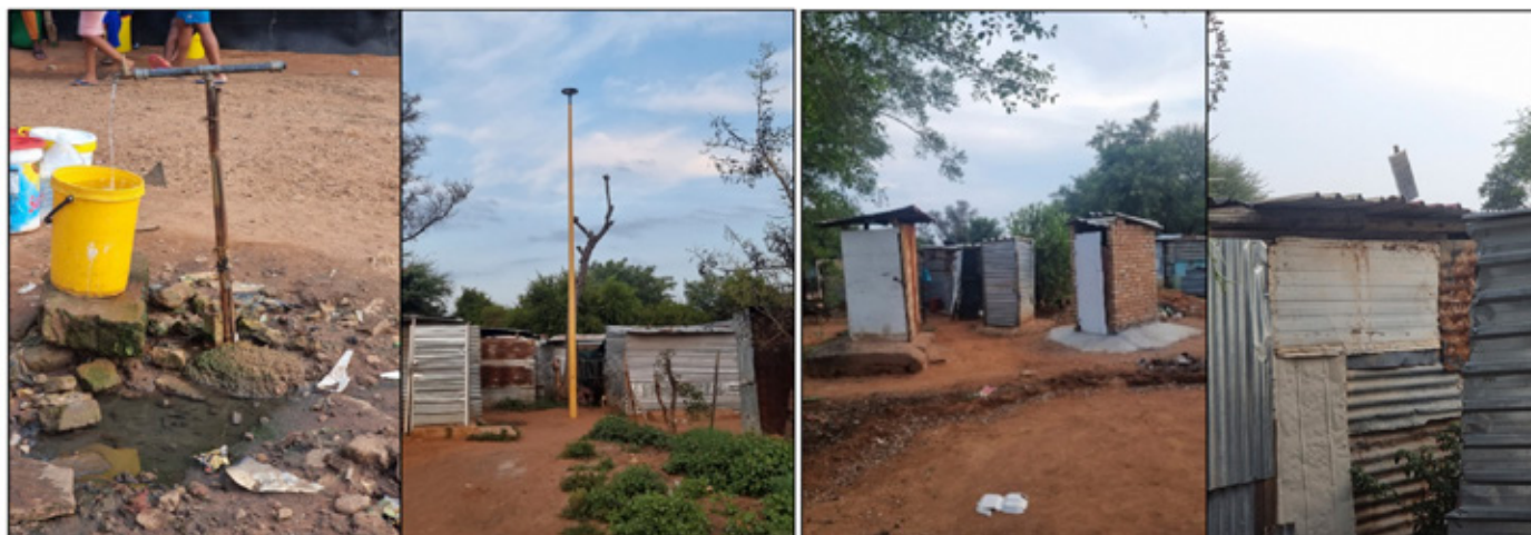
FIGURE 2: Some of the infrastructure available at the Mahlokong informal settlement. The picture on the left shows a communal standpipe (L) and a solar-powered flood light (R) while the picture on the right shows community-built pit latrine toilets (L) and solar panels (R).
