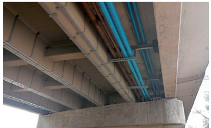
FIGURE 12: Steel plates to the bridge soffits for strengthening
