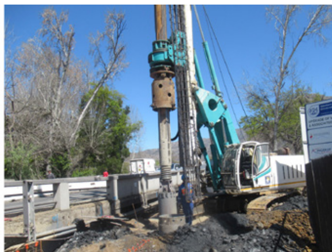
FIGURE 8: ODEX/Rota piles at abutment extensions.
