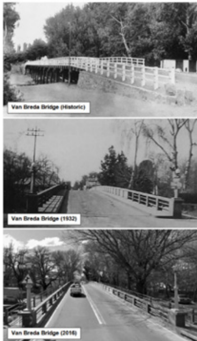
FIGURE 2: Historic Photographic Images of van Breda Bridge
