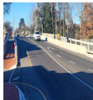
FIGURE 16: Completed bridge and approach road from east
