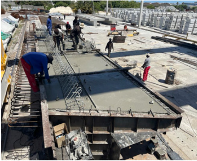
FIGURE 10: Precast beam manufacture
