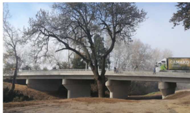
FIGURE 15: Completed bridge (side view)
