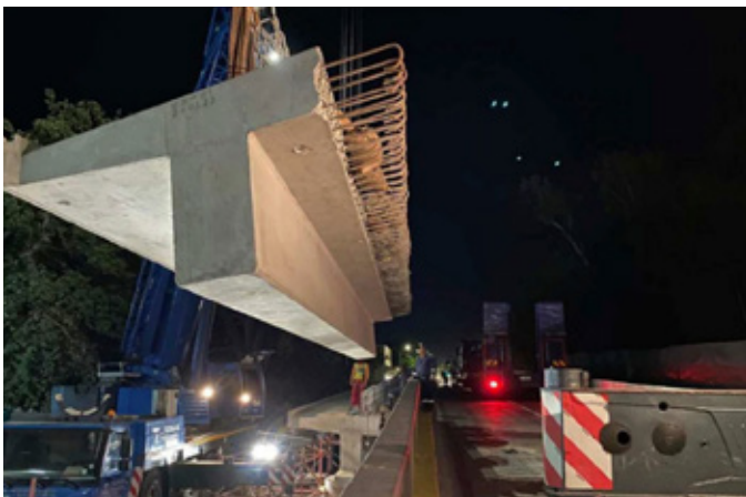
FIGURE 11: Precast T-beam being lowered into position by two mobile cranes
