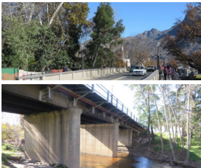
FIGURE 3: Van Breda Bridge (June 2016)
