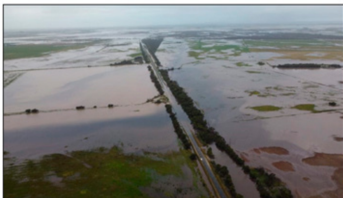
FIGURE 2: Aerial view of flooding along the MR261
