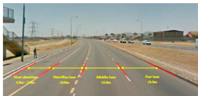
FIGURE 2: Typical northbound carriageway geometry
