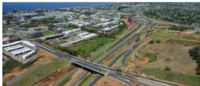
FIGURE 4: Cornubia Bridge linking C9 Route from KwaMashu to Umhlanga (Tongaat Hulett website)
