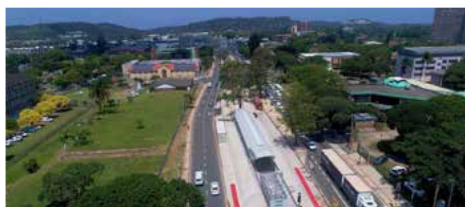
FIGURE 6: ROW Lane on Josiah Gumede Avenue, Pinetown – running east, illustrating the station and station precinct visions of mixed land-use, integration of tactile paving, lateral separation of bus lanes and other traffic modes (Skybox Media)
