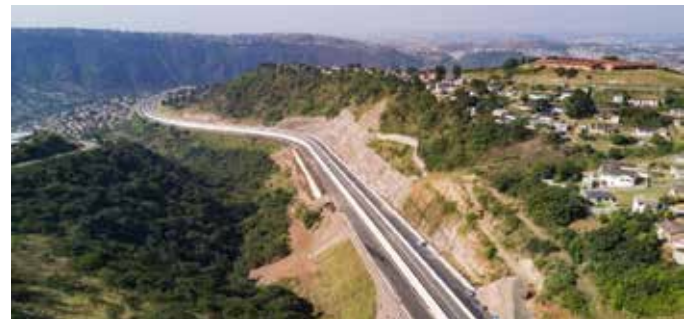
FIGURE 2: MR577 6-lane dual-carriageway, lateral separation between bus lane and other modes of transport. ROW Lanes separated by concrete barrier kerbs on KZN DoT roads (Tongaat Hulett website)
