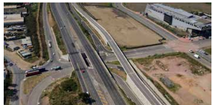
FIGURE 3: M25 Bhejane Underpass linking the C9 Route from KwaMashu to Umhlanga (Go! Durban website)
