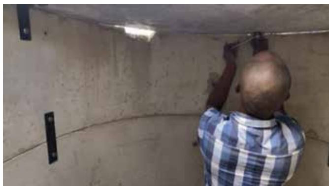
FIGURE 12: installation of internal chamber braces
