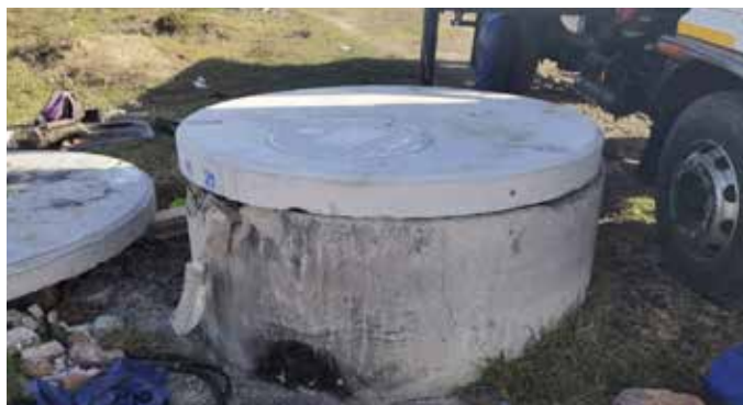
FIGURE 15: Replacement cover slab with smart manhole
