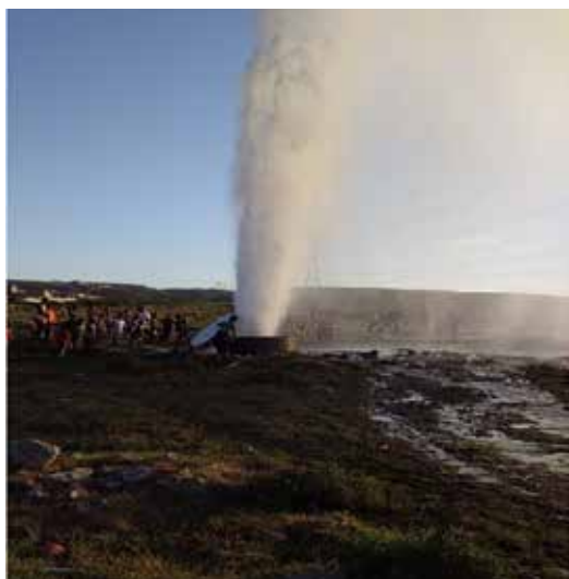
FIGURE 1: Burst as a result of a stolen air valve
