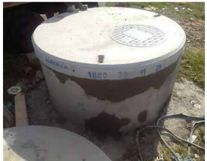
FIGURE 2: Repaired and secured chamber
