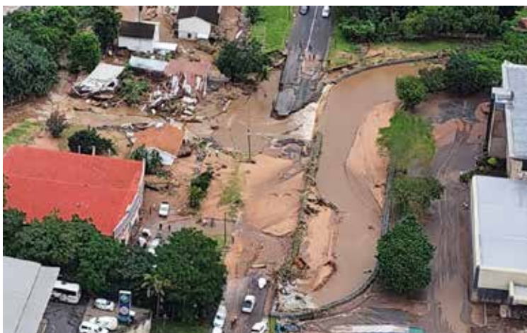
FIGURE 6: Caversham Road damage
