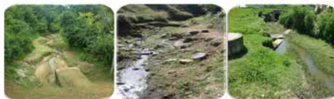
FIGURE 1: Sihlanzimvelo Streams after work has been completed
