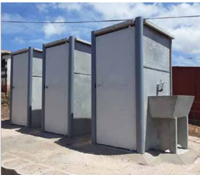
FIGURE 15: Communal Sanitation Facilities: Mosselbay with 5 users to 1 facility
