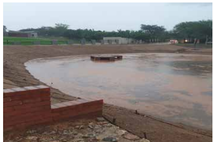
FIGURE 13: Flood events photographic records
