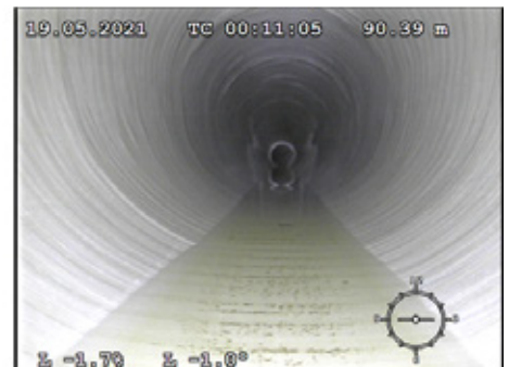
FIGURE 27: 1350mm diameter pipe after rehabilitation with cured in place pipe liner
