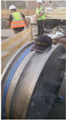
FIGURE 19: Folding packer with strapping bands
