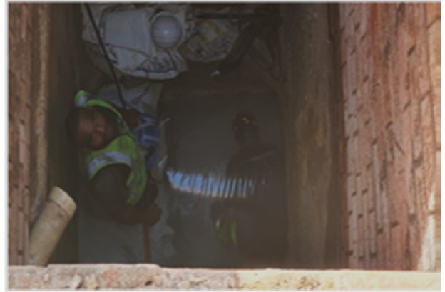
FIGURE 21: CIPPL liner being inflated after packer installed
