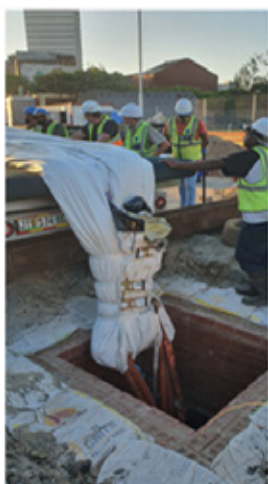
FIGURE 16: CIPPL being inserted into a manhole
