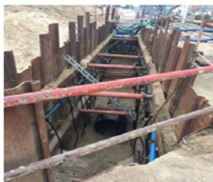
FIGURE 2: Phase 1 open trench construction with deep shoring and dewatering
