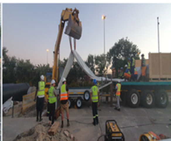
FIGURE 18: CIPPL arriving on site in protective packaging
