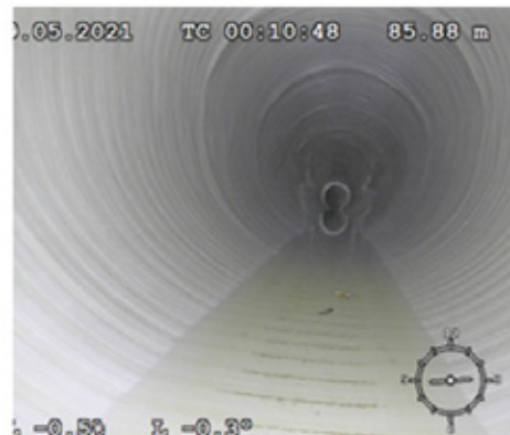
FIGURE 8: Cured in Placed liner cured by UV light on the project
