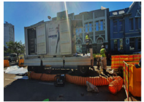
FIGURE 24: UV Rig used to control the curing of the UV Light train
