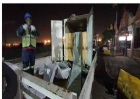
FIGURE 31: CIPP liner arriving on site in refrigerated unit at night
