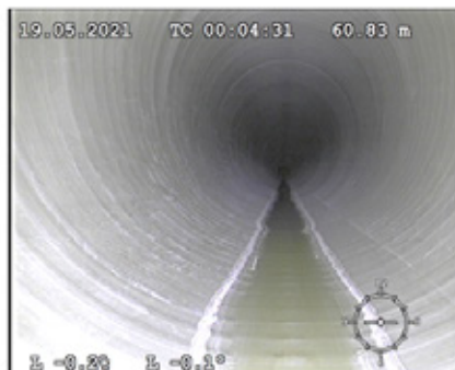
FIGURE 26: 1350mm diameter pipe after rehabilitation with cured in place pipe liner
