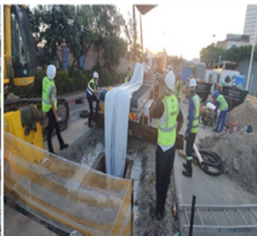
FIGURE 17: CIPPL being inserted into a manhole using a conveyor belt
