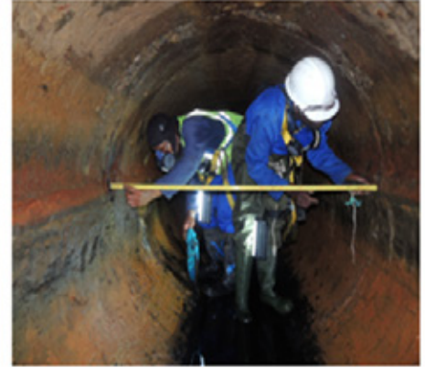
FIGURE 14: Onsite ovality measurement after flow diversion and pipe cleaning
