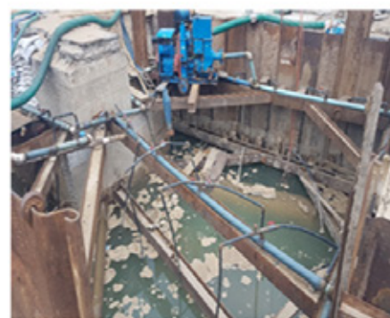
FIGURE 3: Phase 1 open trench construction with high water table below sea level
