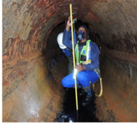
FIGURE 12: Onsite ovality measurement after flow diversion and pipe cleaning
