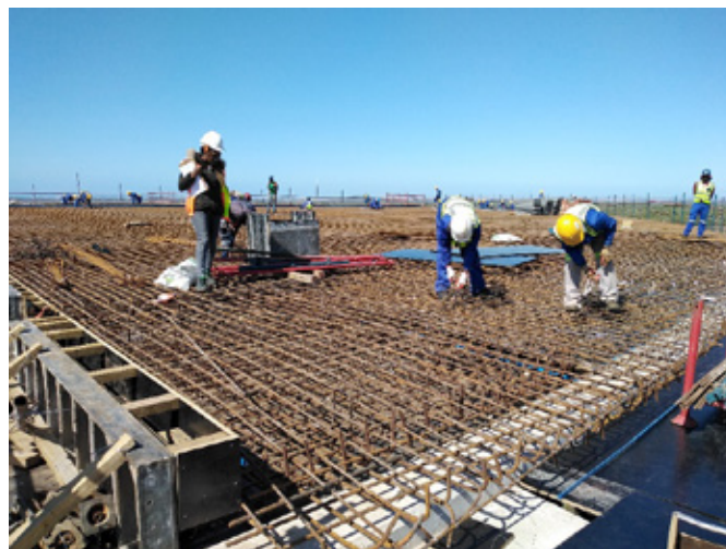
FIGURE 3: Nooitgedagt WTW - EME's assisting with steel fixing.
