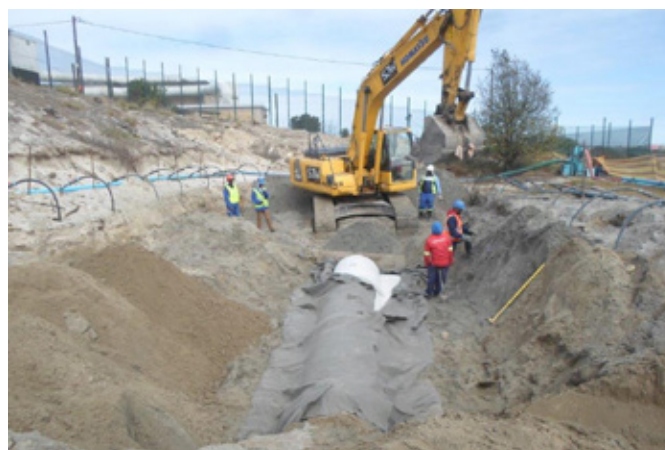
FIGURE 4: Markman Sewer - EME's assisting with pipe laying operations.
