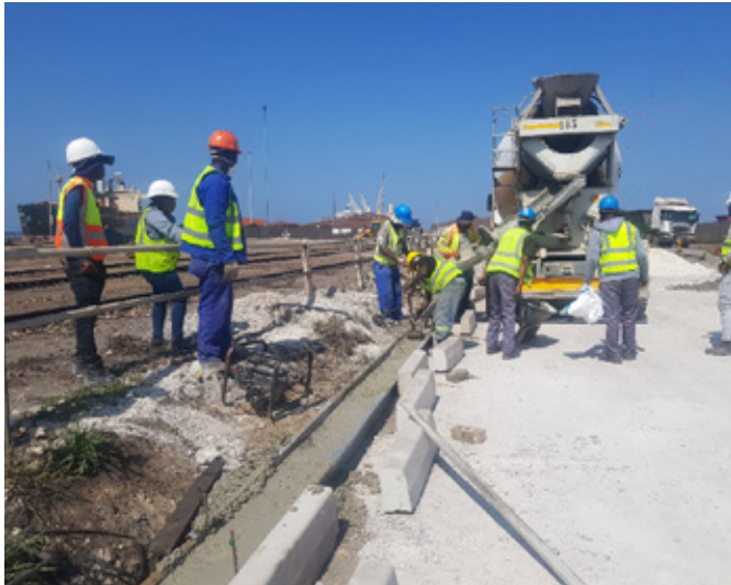
FIGURE 5: Flemming Road - EME's laying kerbs.
