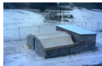
FIGURE 8: Emergency dosing facility at Grassridge
