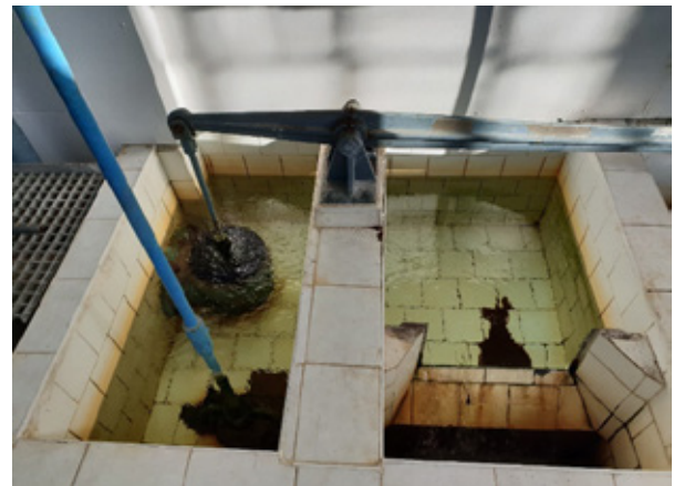
FIGURE 4: Filter module before refurbishment
