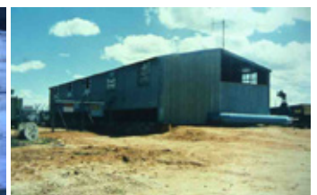
FIGURE 9: Emergency pump station at Nooitgedagt
