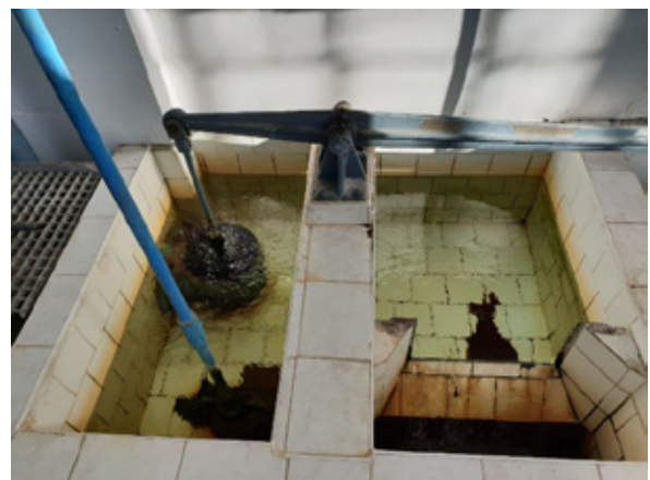
FIGURE 5: Filter modules after refurbishment
