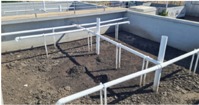
FIGURE 8: Faecal sludge drying beds at a Faecal Sludge Treatment Plant in Shinyanga, Tanzania
