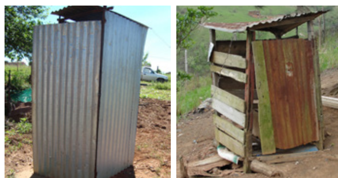
FIGURE 3: Typical unimproved pit latrines, built from cheap or freely available materials. While these toilets are generally unpleasant and sometimes unsafe to use, they do not present a faecal sludge management challenge. When the pits are full the structures are moved and the pits are covered.
