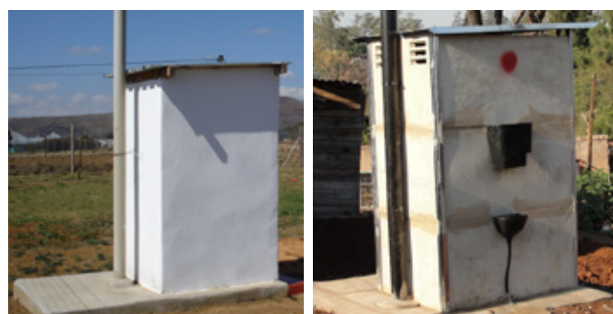
FIGURE 4: Ventilating Improved Pit Latrines (VIPs) in South Africa are typically of masonry or precast concrete construction. In the last 10 years the latter type has become standard, due to their speed and ease of construction. To ensure stability the underlying pits must be partially or preferably fully lined. The pits should not, however, be sealed, as that will turn the pits into conservancy tanks which require much more frequent emptying.
